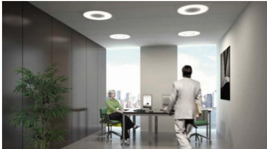
Fig. 4. Philips DayZone luminaire (system) in an office application. One of the earliest functional LED office luminaires applied in a ceiling. Luminaires at window side are switched on in the 500 lux setting, the two luminaires in front are switched on according the 300 lux setting.
