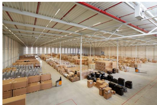
Fig. 7. Typical application of light line systems in industry. Long (semi-) continuous lines of light illuminate the area.
